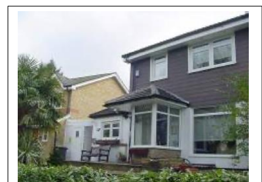
How vertical tiling and new windows can considerably change the look of a property but underneath it is still a metal framed building
