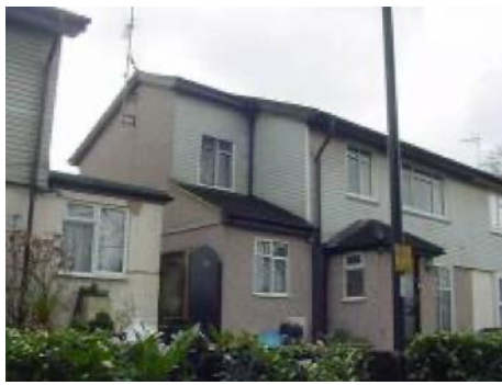
Pebbledash render in parts as well as plastic cladding and extensions but again the main part of the building is still a metal frame
