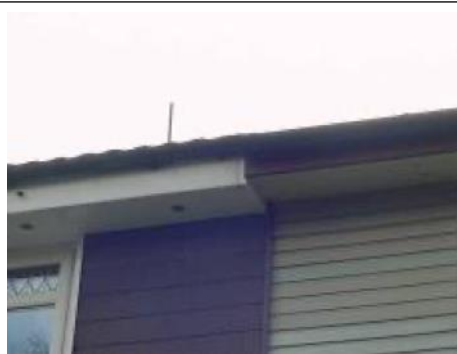
Example of plastic overcladding
