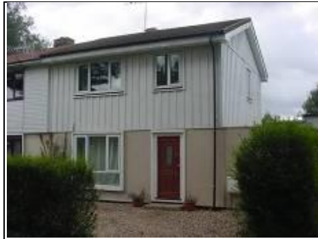
Example of BISF house with metal cladding at high level and render at low level (Not your property)
