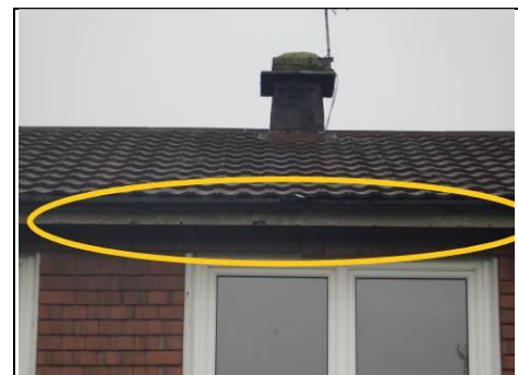
Fascias and soffits
