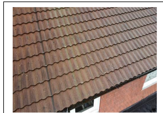
Pressed metal tiles to rear
