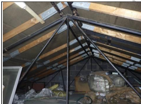
Tubular metal structure in roof
