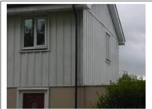
Originally the property would have had profile metal cladding
