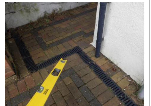
Front right downpipe feeds directly into ground
