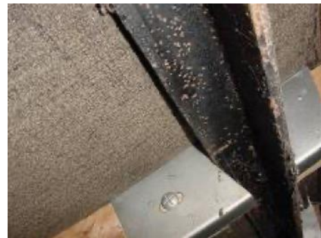
Some fixings replacements/repairs to a non-traditional house
