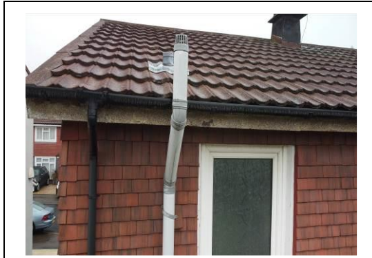
Relatively new plastic soil and vent pipe
