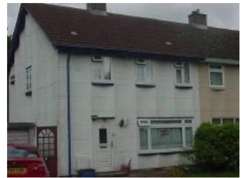
Non-Traditional house mainly asbestos
