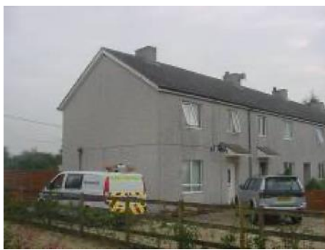
Large panel concrete non-traditional house
