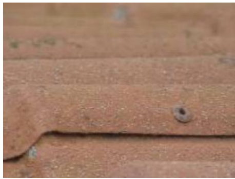
Rivet where you can see roof is riveted together
