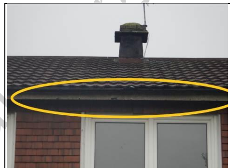
Fascias and soffits
