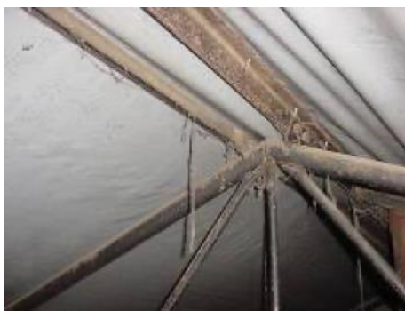
Example of tubular metal frame within the roof of a metal framed property
