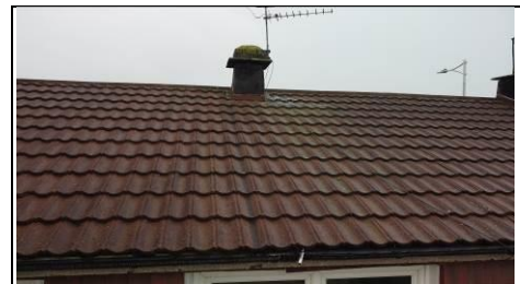
Pressed metal roof Aerial view
