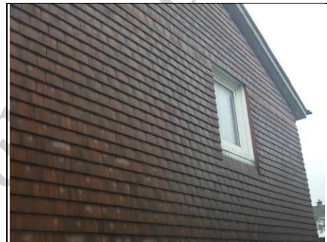
Vertical tiling to right gable
