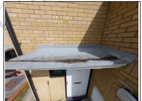
Front entrance canopy
