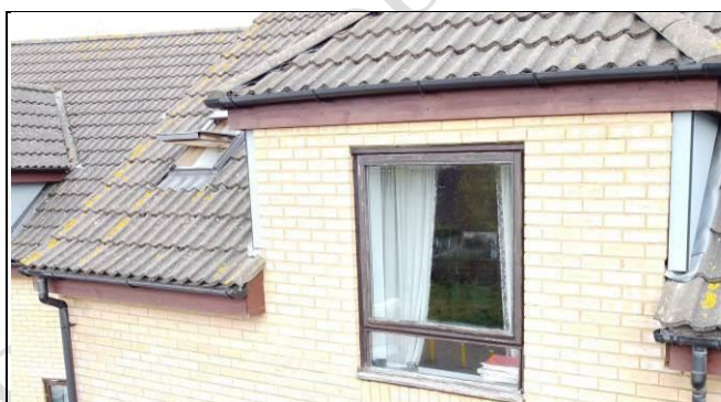
Fascias and soffits ~ Aerial View - 360 Photo ~
