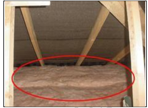
Roof insulation in modern property
