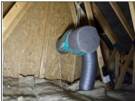
Left gable plywood
