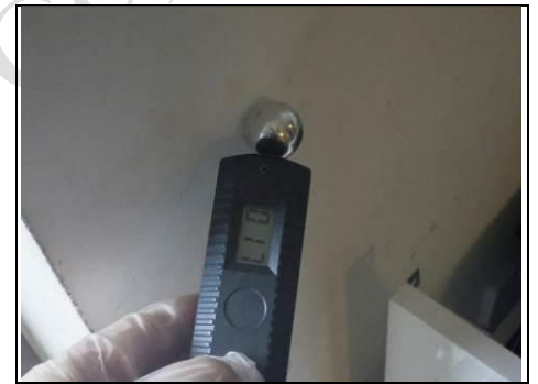
Testing for lateral dampness
