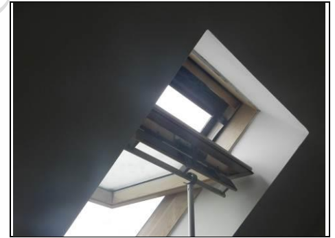
En-suite roof window open at time of survey
