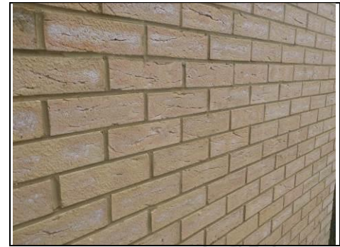
Efflorescence
