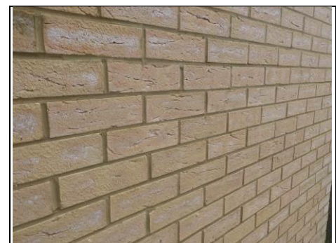
Efflorescence
