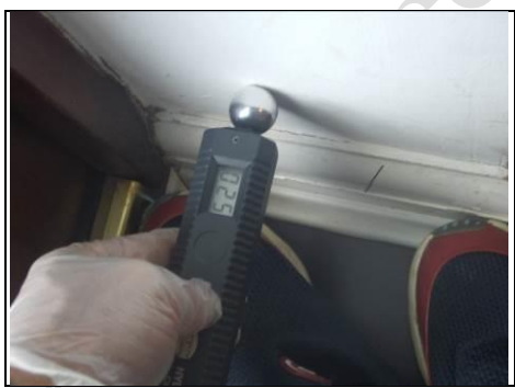
Testing for rising damp
