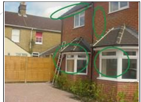
Double glazed windows and loft insulation in modern property
