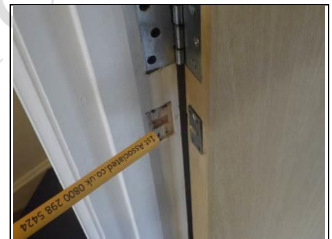
Door closer removed
