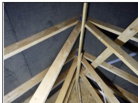
General view of inside of roof
