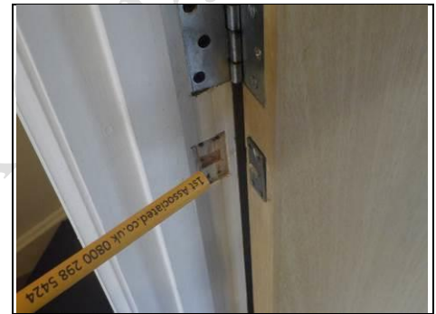
Door closer removed
