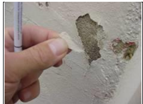
Plastic/polymer based paint on hard cement render
