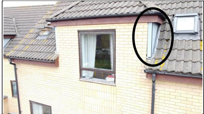
Front dormer timber frame ~ Aerial View - 360 Photo ~
