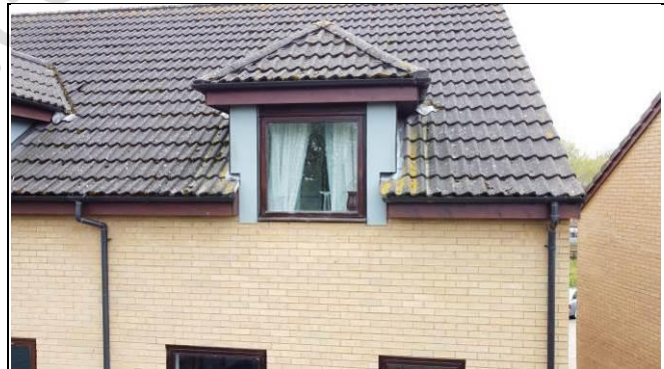
Rear dormer ~ Aerial View - 360 Photo ~
