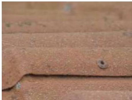
Rivet where you can see roof is riveted together
