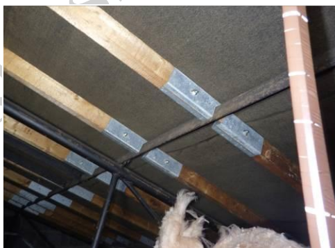
Common rafters with metal sections
