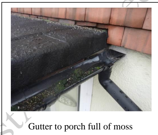
Older style plastic gutters that fade with sunlight
