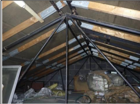
Tubular metal structure in roof
