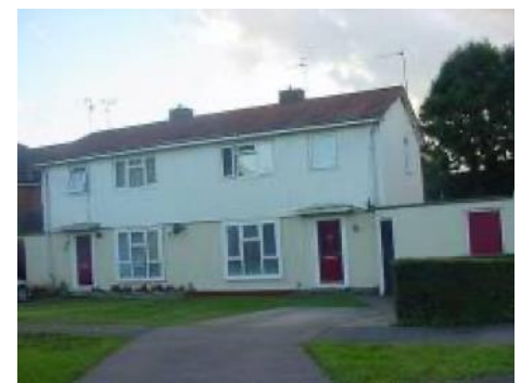
British Iron and Steel Federation frame house (BISF)
