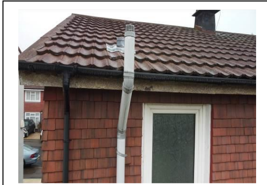
Relatively new plastic soil and vent pipe
