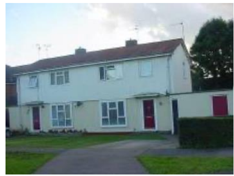
Plastic cladding has been put on top of property
