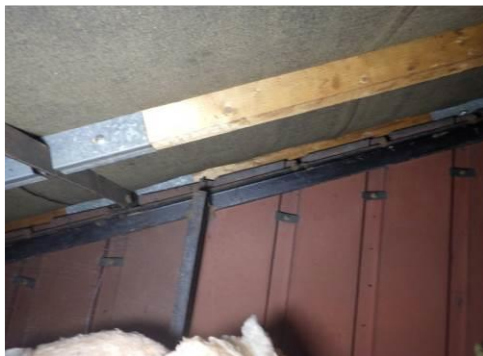
Old external ribbed metal cladding
