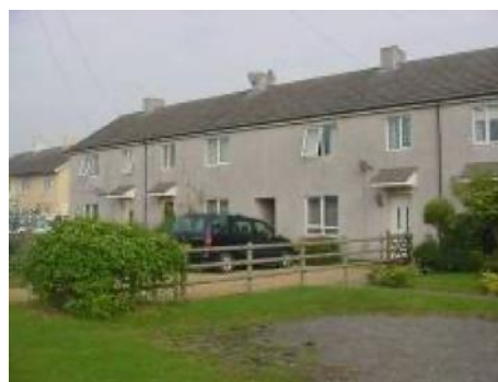
General view of a development of non-traditional houses
