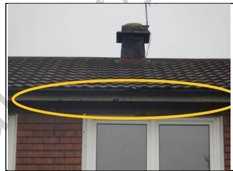
Fascias and soffits
