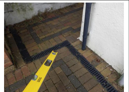
Front right downpipe feeds directly into ground
