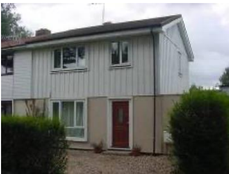
Metal frame house with profile metal sheeting at top and render at bottom. Roof has been changed.
