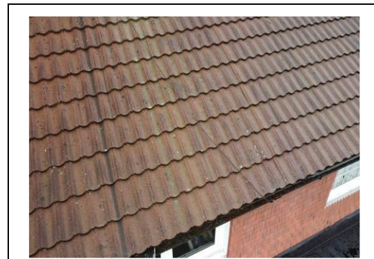
Pressed metal tiles to rear
