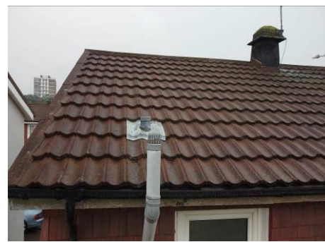
Old capped off soil and vent pipe to rear right
