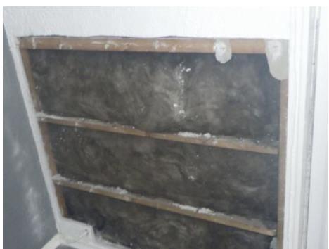
Opening One ground floor hall next to entrance door
