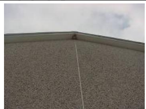
Jointing to a non-traditional house
