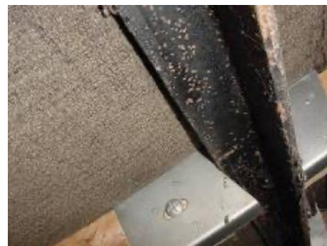
Some fixings replacements/repairs to a non-traditional house
