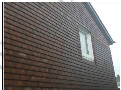
Vertical tiling to right gable
