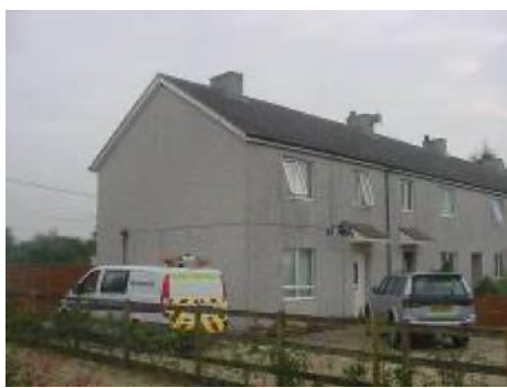
Large panel concrete non-traditional house
