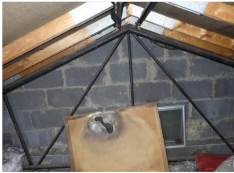
Tubular metal frame and timber common rafters
