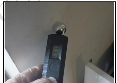
Testing for lateral dampness
