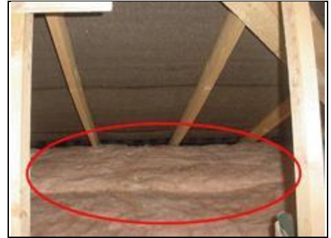
Roof insulation in modern property
