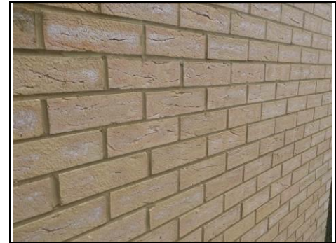
Efflorescence
