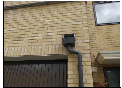
Hopperhead to balcony
