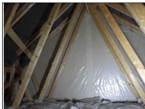
Plastic sheet to right gable
