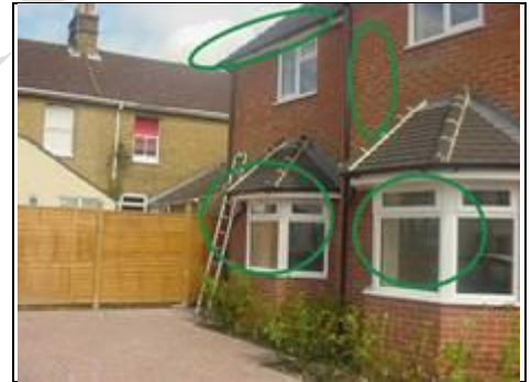
Double glazed windows and loft insulation in modern property
