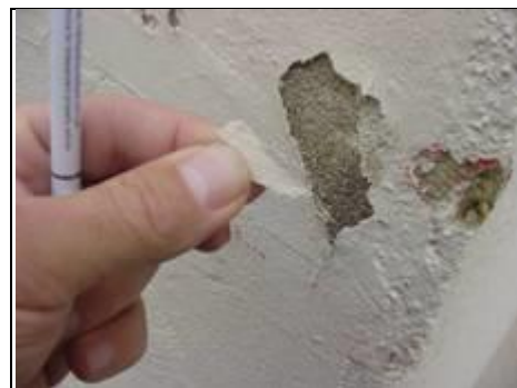
Plastic/polymer based paint on hard cement render
