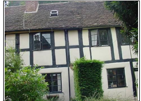
Example of traditional timber frame
