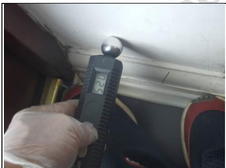
Testing for rising damp
