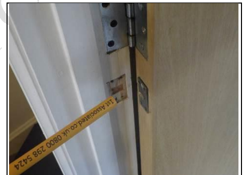
Door closer removed
