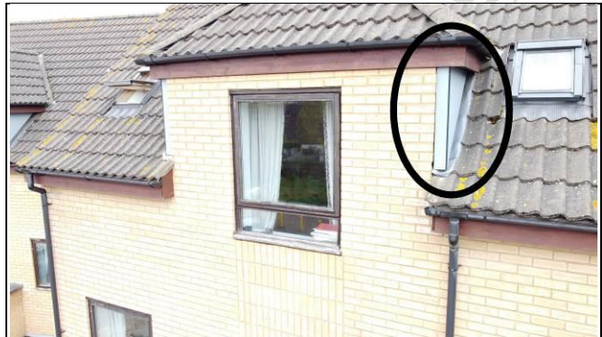
Front dormer timber frame ~ Aerial View - 360 Photo ~
