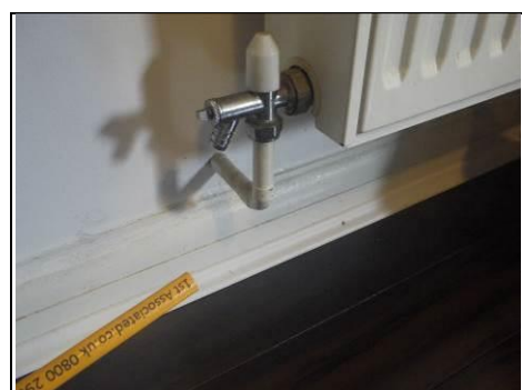
Microbore pipes
