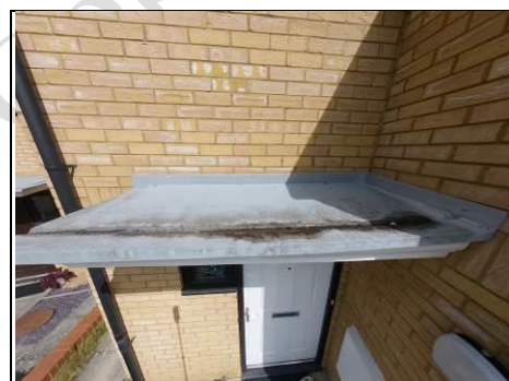
Front entrance canopy
