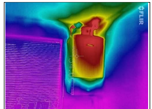
Boiler (Not your property)
