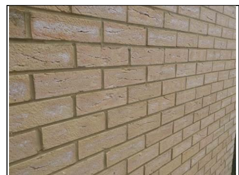
Efflorescence
