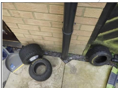
Downpipes feed directly into ground rear left corner
