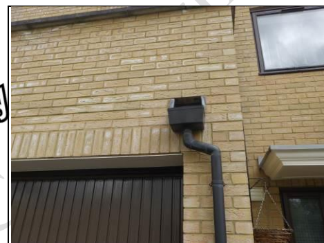
Hopperhead to balcony
