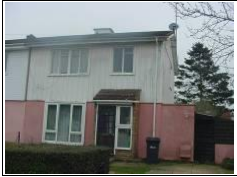
Painted cladding to non-traditional property
