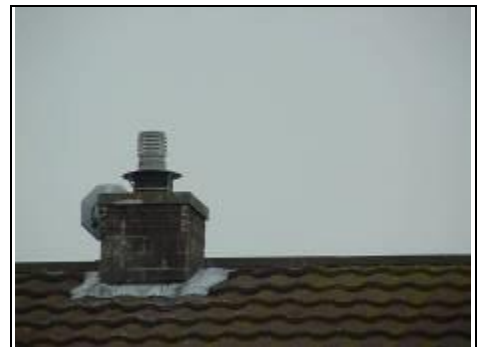
New chimney on a non-traditional house
