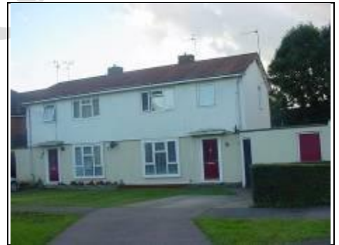
British Steel frame house (BISF)
