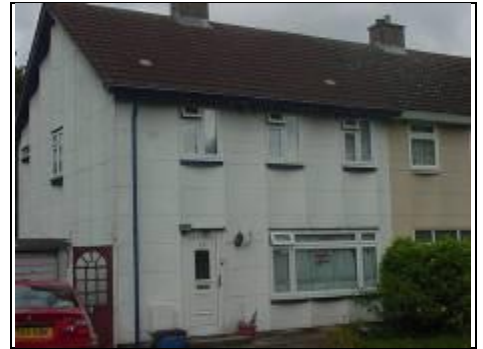
Non traditional house mainly asbestos
