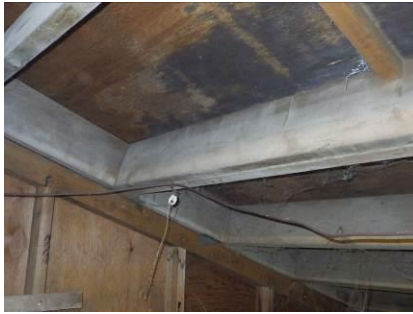
Mould to roof
