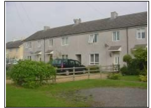
General view of a development of non-traditional houses
