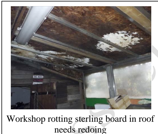
Workshop roof deteriorating, partly replaced with metal profile sheet
