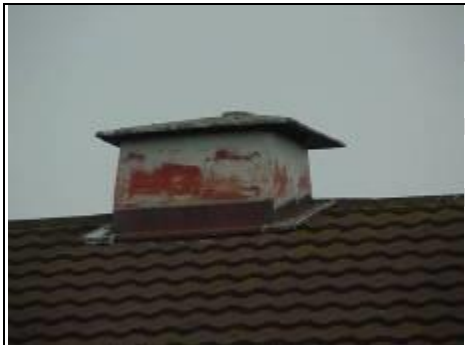
Asbestos original chimney non traditional house
