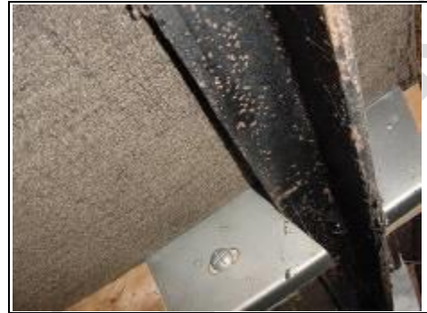
Some fixings replacements/repairs to a non-traditional house
