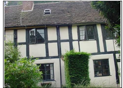
Example of traditional timber frame
