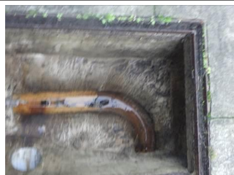
Manhole four near path leading to bar and pool area
