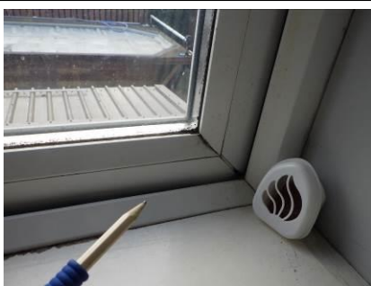
Black mould around window
