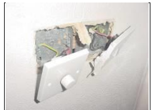
Removing electric points to view construction
