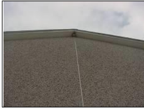
Jointing to a non-traditional house
