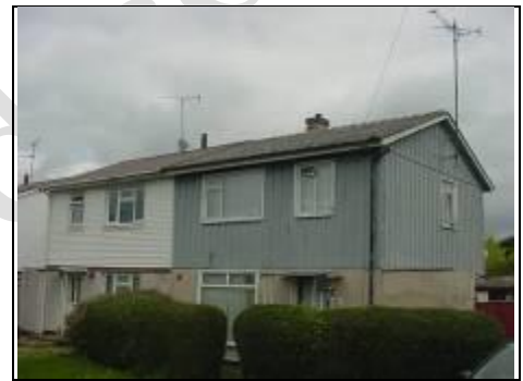
Asbestos roof on BISF house
