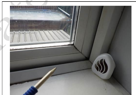
Black mould in shower room
