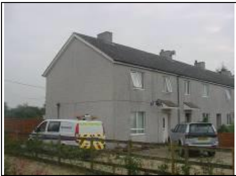
Large panel concrete non-traditional house
