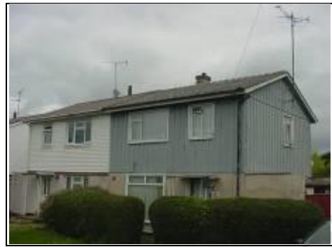
Asbestos roof on BISF house
