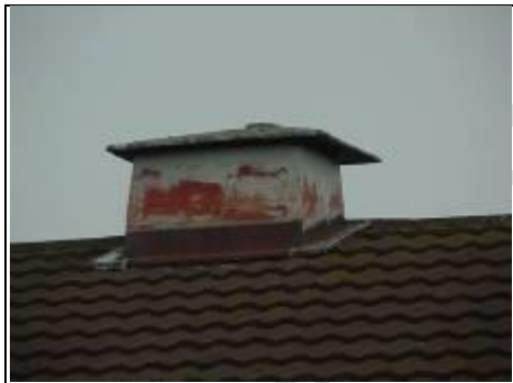
Asbestos original chimney non traditional house
