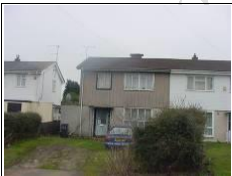
Original condition of non-traditional house with roof replacement
