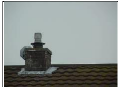
New chimney on a non-traditional house
