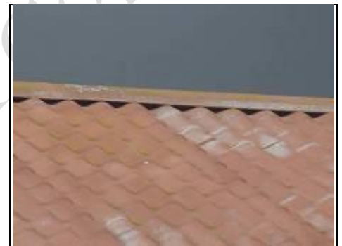
Metal cladding roofs
