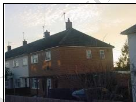
Brick cladding and other alterations make a non traditional house mortgageable
