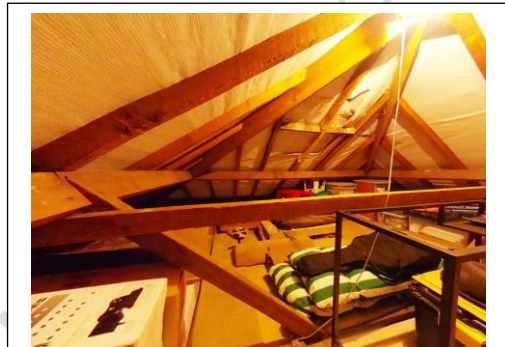
Roof space removed chimney
