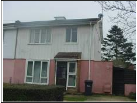
Painted cladding to non-traditional property
