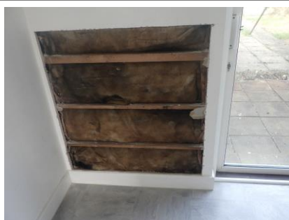
Opening Two next to rear sliding door (Not your property)
