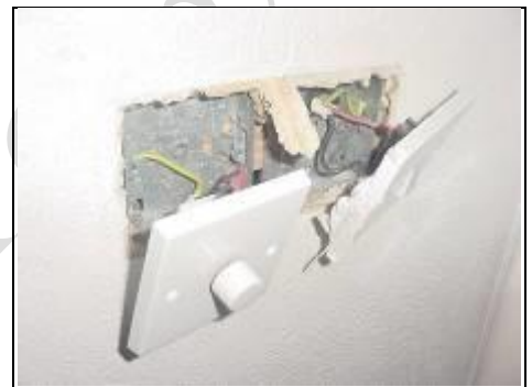
Removing electric points to view construction
