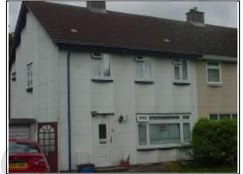
Non traditional house mainly asbestos
