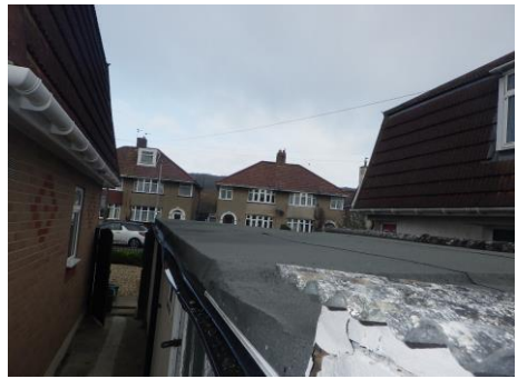
Outbuilding roof basic with felt tacked on
