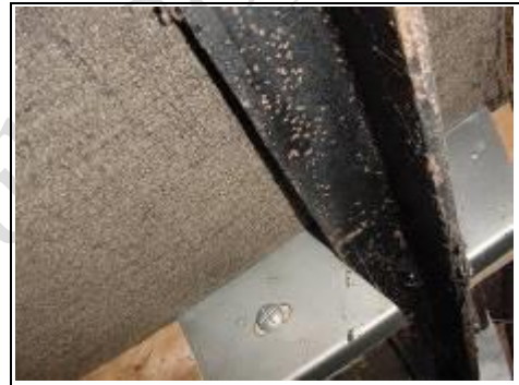
Some fixings replacements/repairs to a non-traditional house
