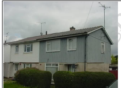
Asbestos roof on BISF house
