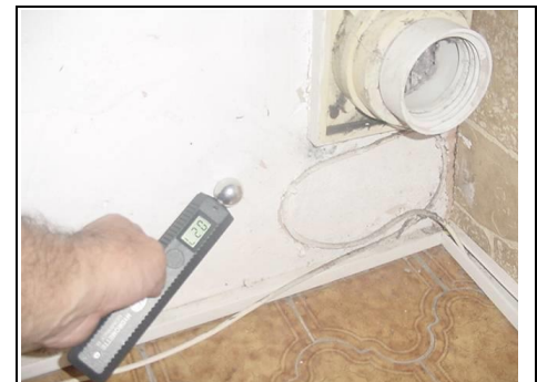
Testing for rising damp
