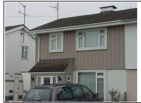
Non-traditional metal frame house
