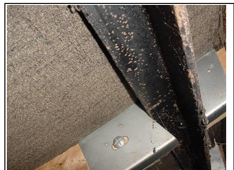
Some fixings replacements/repairs to a non-traditional house
