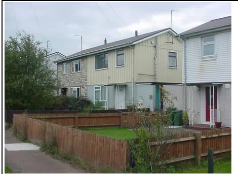
British Iron and Steel Federation House (BISF)
