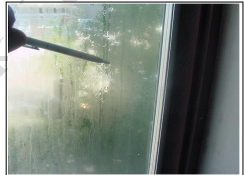
Misting over to front double glazed window
