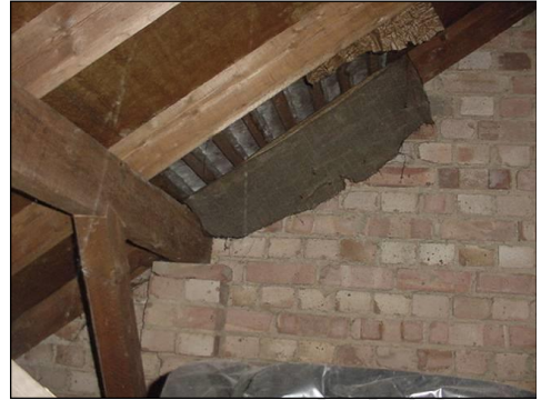
Brick firewall, which is a party wall
