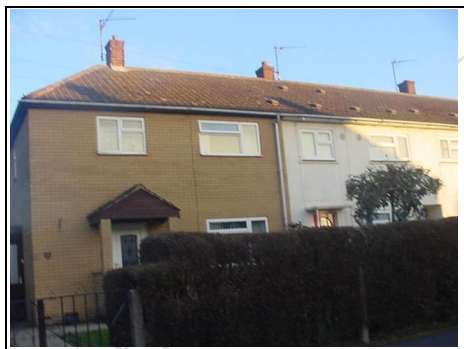
Brick clad modified non traditional house
