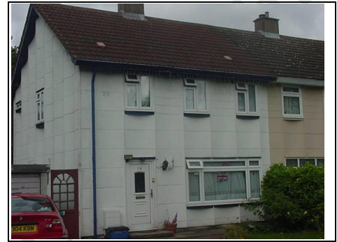
Non traditional house mainly asbestos
