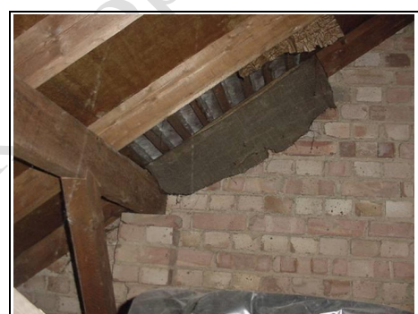
Purlin sits on brickwork
