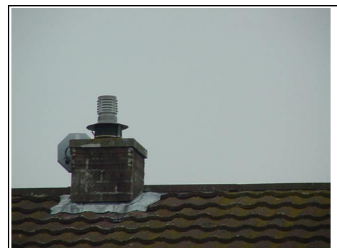
New chimney on a non-traditional house
