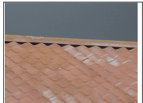
Metal cladding roofs
