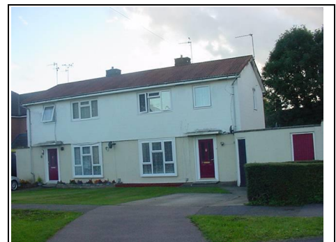
British Steel frame house (BISF)
