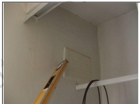
High level airbricks
