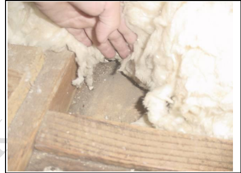
Plasterboard/proprietary boarding underneath insulation
