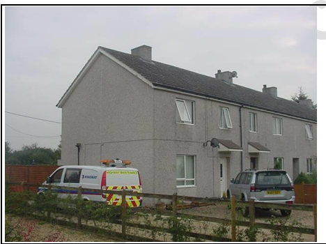
Large panel concrete non-traditional house
