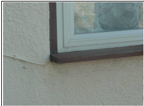
Older style double glazed windows within timber frame
