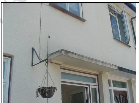
Front concrete canopy roof
