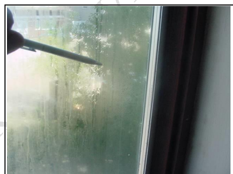
Misting over to front double glazed window
