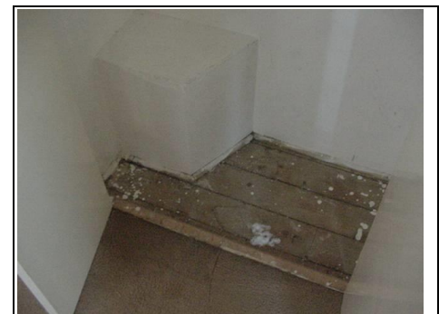
Floorboards – joists run from front to rear of property
