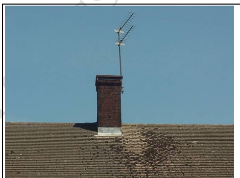
Rear view of chimney
