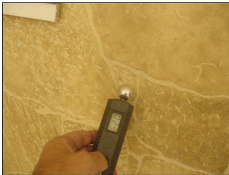
Testing for lateral dampness onto a dry-lined wall
