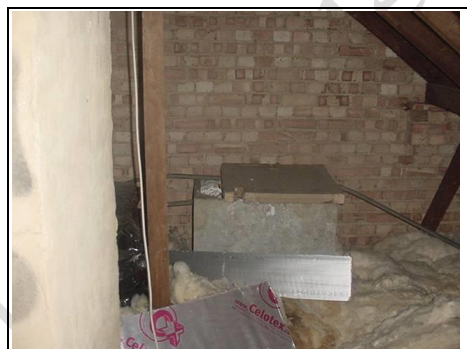
Old cast iron water tank still in roof
