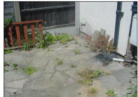
General undulations in crazy paving to rear
