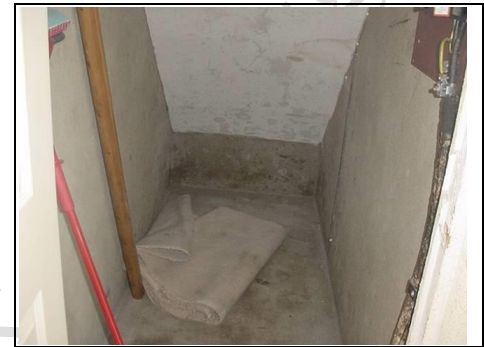
Concrete visible under stairs
