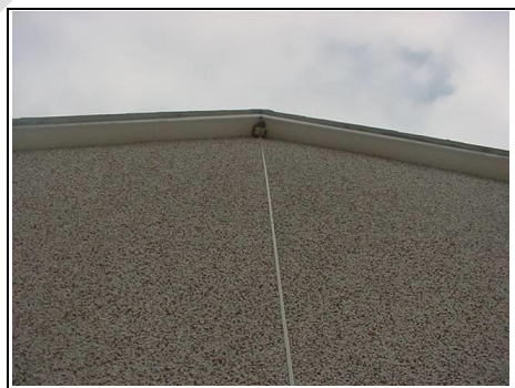
Jointing to a non-traditional house
