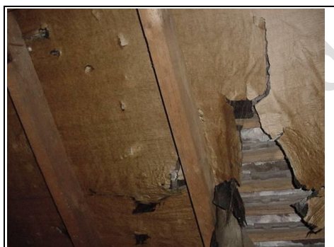
Older style building paper in roof
