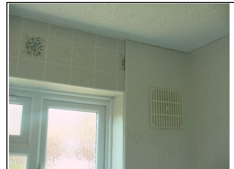
Sliding vent sometimes known as a hit and miss vent
