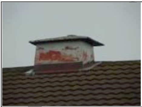
Asbestos original chimney non traditional house
