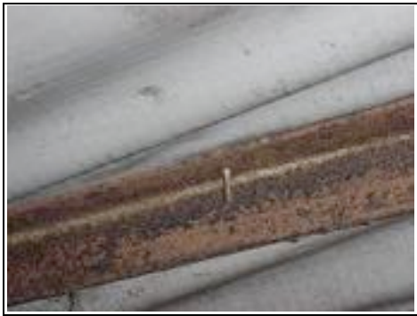
Example of excessive rusting that we have seen in the roof of a metal framed building compared with the rusting in your house which is less than this
