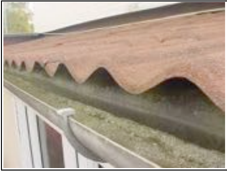
Close up of edge of profile metal roofing that looks like a tile
