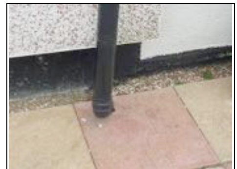
Downpipes feed directly into the ground
