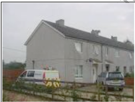
Large panel concrete non-traditional house
