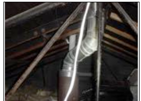
New flue for boiler
