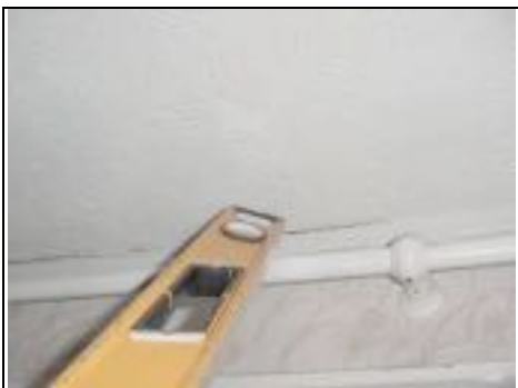
Cracks corner of walls to ceiling
