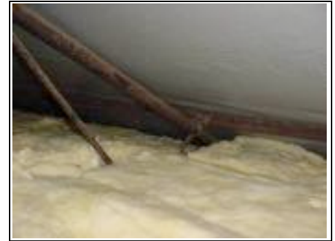
Example of over insulation of a metal framed property which causes condensation
