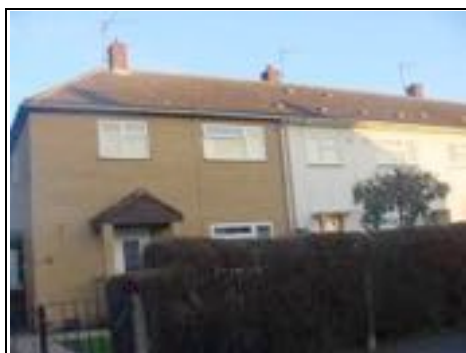
Brick clad modified non traditional house
