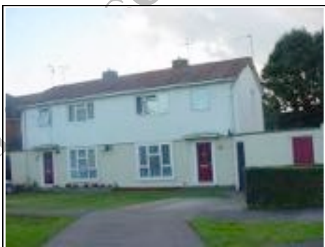
Plastic cladding has been put on top of property
