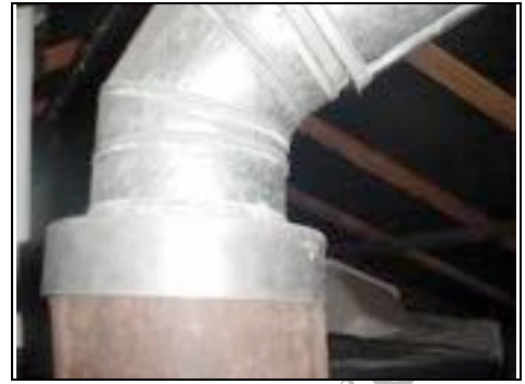
Flue possibly asbestos
