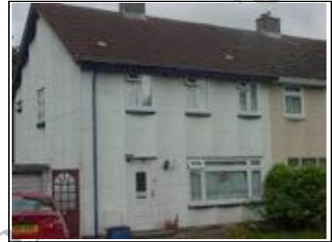
Non traditional house mainly asbestos
