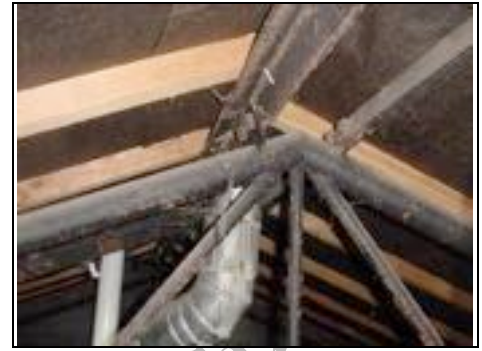
Tubular roof system and timber batons
