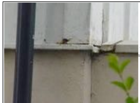
Rusting to profile metal cladding
