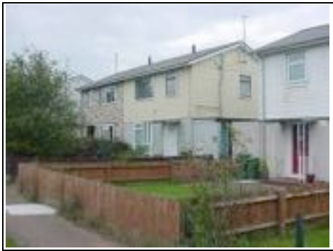
British Iron and Steel Federation House (BISF)
