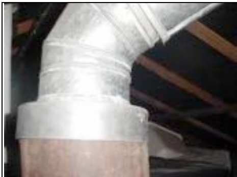
Possible asbestos to flue
