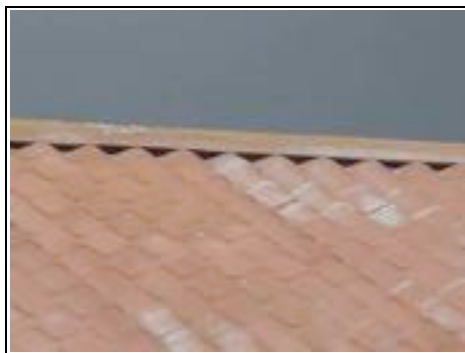
Weathering effect to roof
