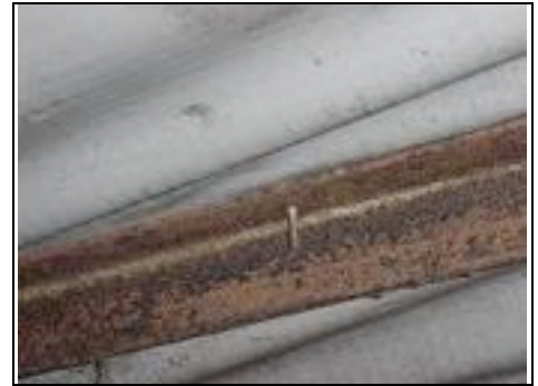
Example of what we would term as excessive rusting on another property
