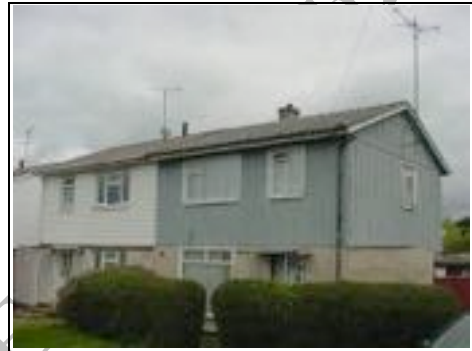
Asbestos roof on BISF house
