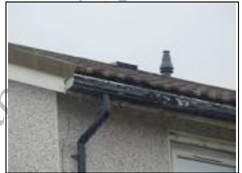
Metal gutter and plastic downpipe
