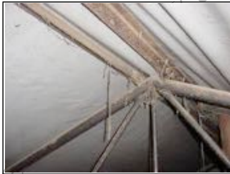
Example of tubular metal frame within the roof of a metal framed property
