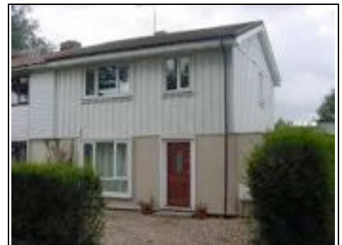
Originally the property would have had profile metal cladding as per this example
