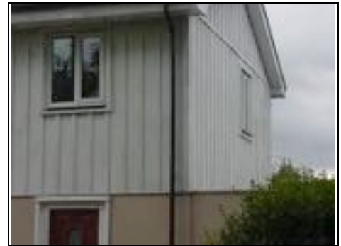
Example of metal cladding on a BISF house
