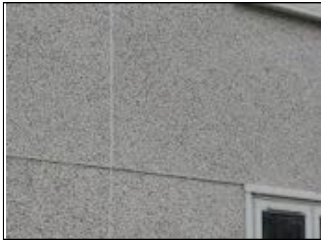
Movement joints within the panel construction that have been added
